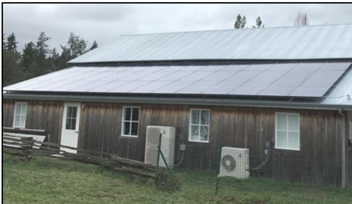
Rain Shadow Solar from Orcas Island installed 36 solar panels on the roof of the MHI. Let the sun shine!
