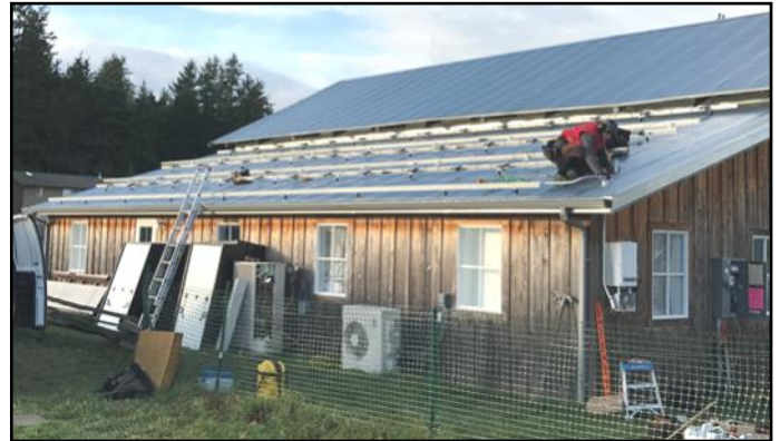
Mounting grids being installed on the roof of the MHI.
