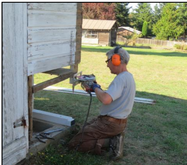
During: Contractor Alan Smith working his magic.
