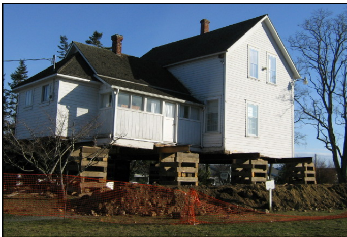
King house awaiting a new foundation
