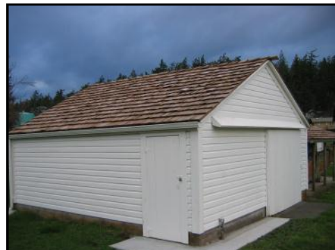
Carriage House after
