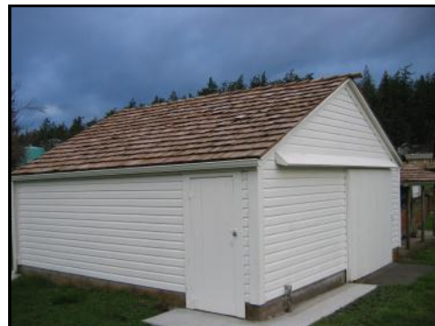
Carriage House after
