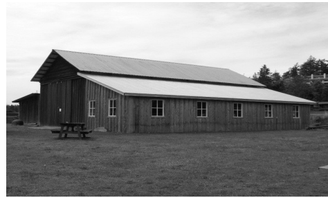
The remodeled south side of the barn
